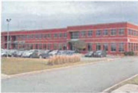
Fig. 72 ADT Security Services et Johnson Controls (Source: Google Street View, 2016)
