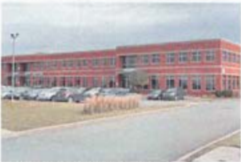
Fig. 72 ADT Security Services et Johnson Controls (Source: Design Total Plus, 2016)
