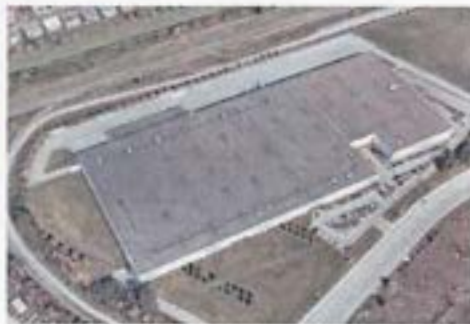
Fig. 73 Centre de distribution Belmans (Source: Design Total Plus, 2016)
