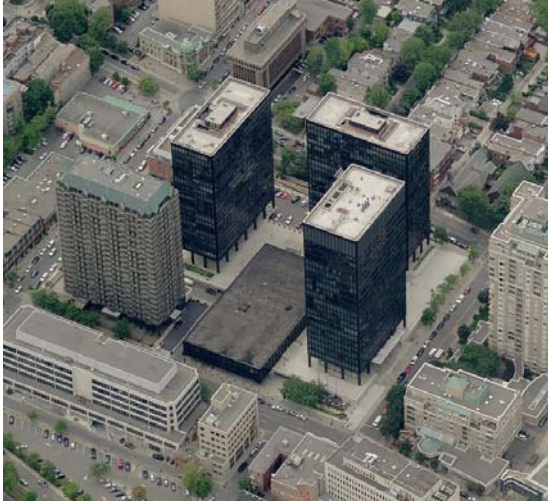
Aerial view: Source: Bing Maps
