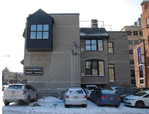
Rear (East) Façade
