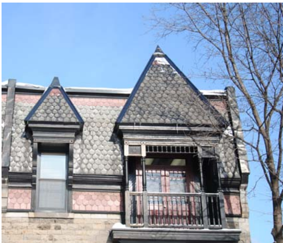
Detail of the Mansard Roof
