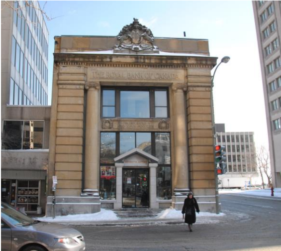
North (Front) Façade: Ste-Catherine Street West
