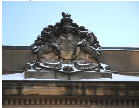
Front Facade Insignia at the Top of the Parapet
