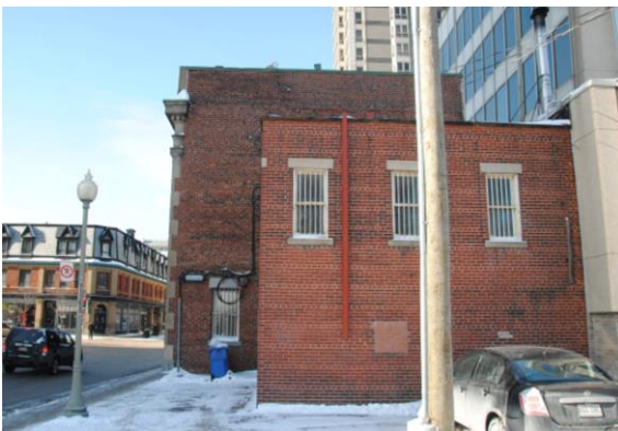
South (Rear) Façade
