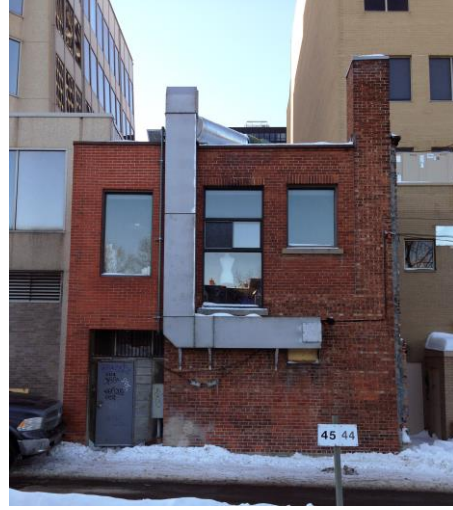
South (Rear) Façade
