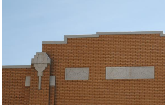
Front Façade: Details of the Cast Stonework, Featuring Art-deco Geometric Patterns
