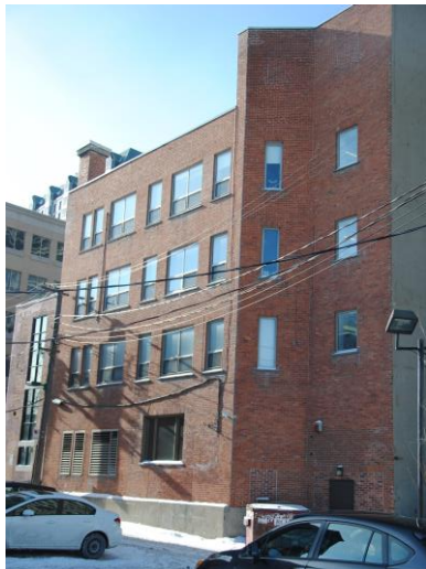
South (Rear) Façade
