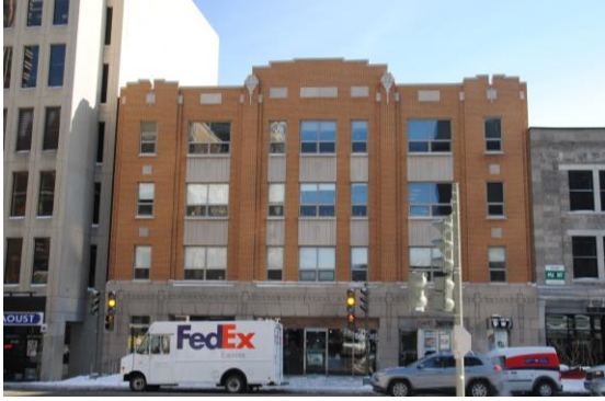
North (Front) Façade
