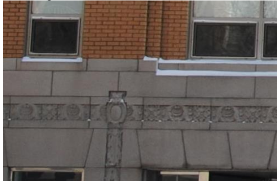
Front Façade: Details of the Cast Stonework on the Building Base
