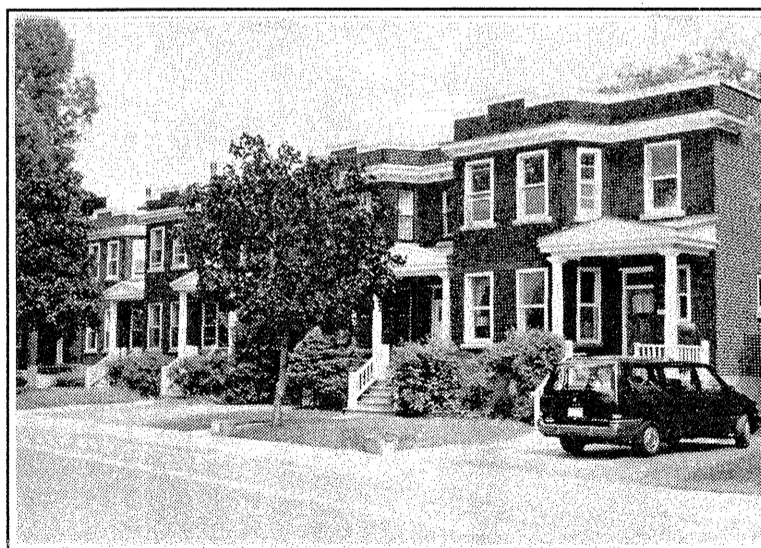
De Maisonneuve Blvd., south side: wood porches with pediments, bay windows and cornices.
