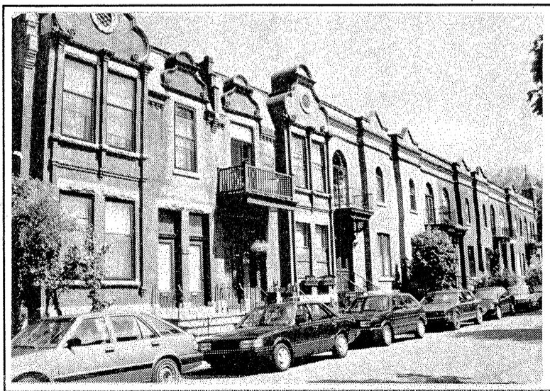
Winchester Ave., north side: bay projections, balconies and articulated parapets.
