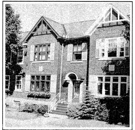
Parkman Place, south side: vertical windows in horizontal openings, shutters and entrances with canopies.
