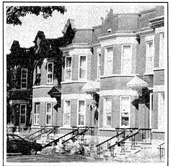
Windsor Ave., south side: two-storey bay windows, entrance canopies and articulated parapets.
