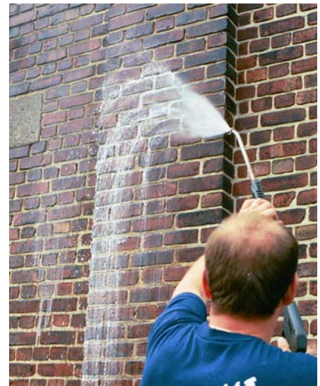
Only the gentlest methods should be used to clean masonry walls.
