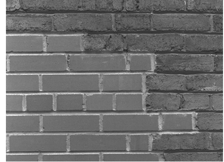
When repointing part of a wall, avoid using a new mortar that does not match the existing in color and details.
