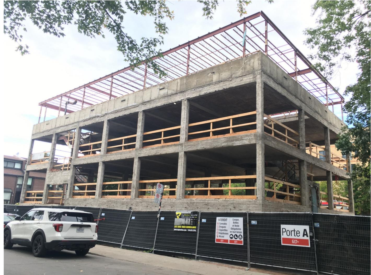
Under the approved Site Planning and Architectural Integration Program (SPAIP), less than 50% of the exterior walls and roof of the building were to be demolished. However, at the time of the work, it was found that the building envelope was damaged. Consequently, more than 50% of it was demolished.
