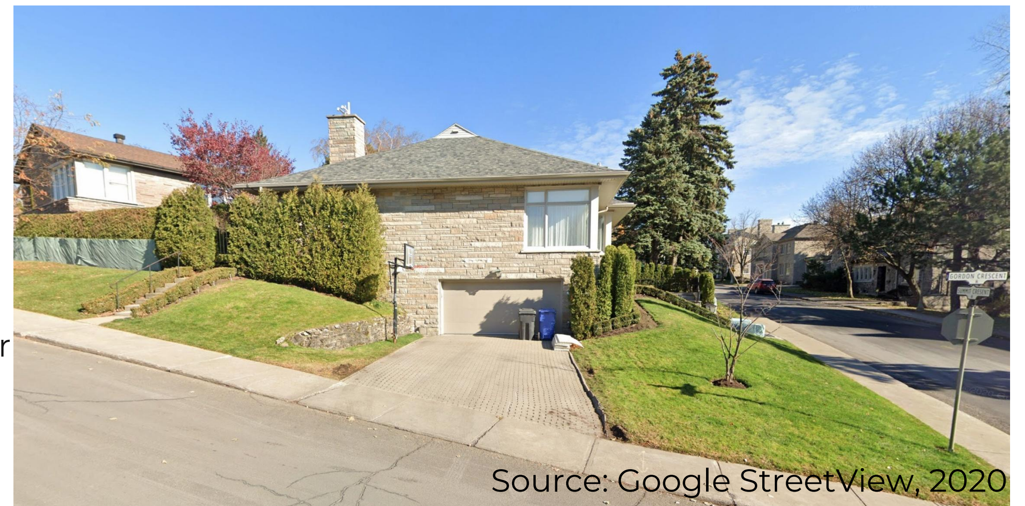
Side façade on Gorden Crescent
